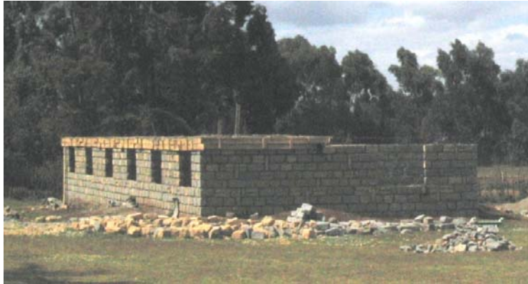
Medical Clinic under construction
